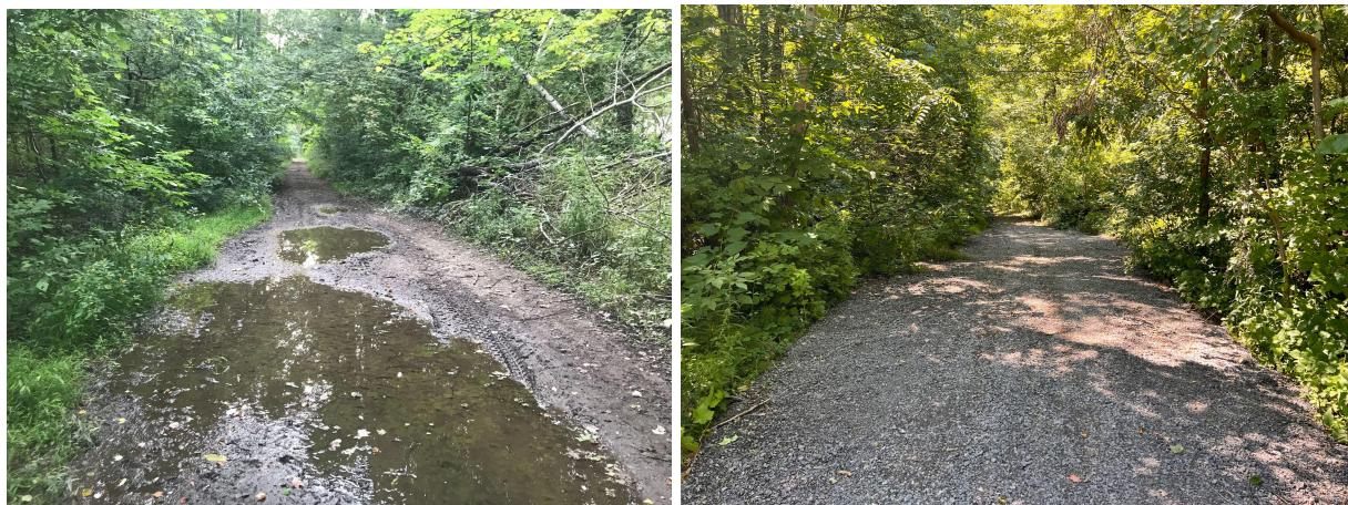
The pictures below show the before and after of the Nadine and Paul Webb Trail near Morris Road in Mayville. Numerous drainage and reditching work was done to begin the improvement of that section. Especially in the spring and fall, the section used to have numerous puddles.
