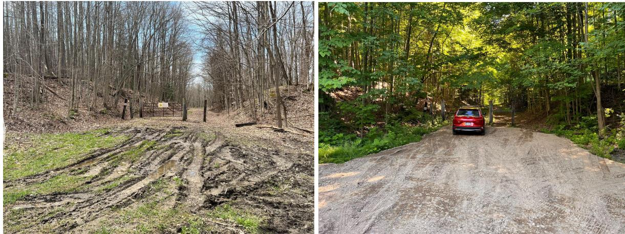
Also, on the Ralph C. Sheldon Jr. Trail near Nettle Hill Road, the pictures below show the before and after of the work that was done. The area was reditched to improve the drainage of the chronically wet section, and the part of the trail near the road was resurfaced.
